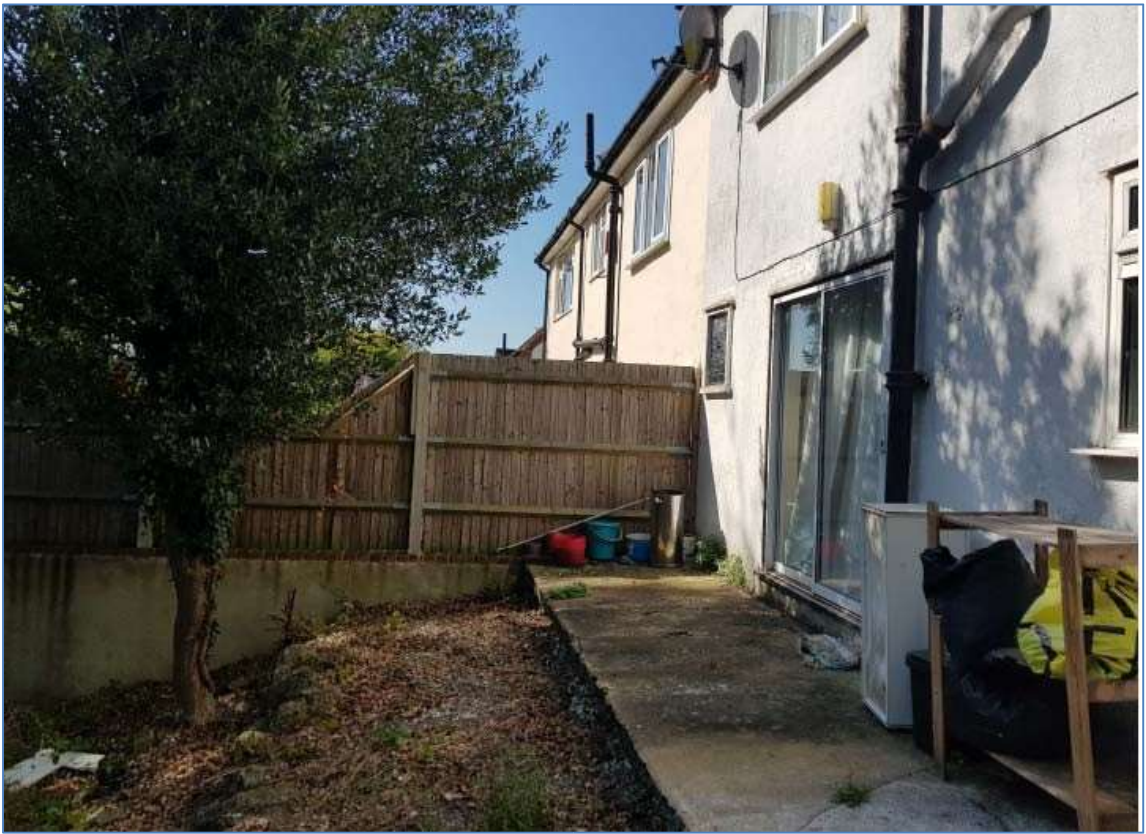
Figure 2: Side boundary with a high fence
